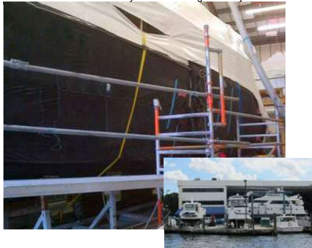
Surface treatment of luxury boat hull using flexible jackets
