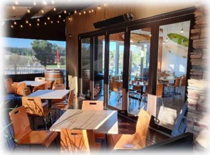
DINING AREA – PANEL HEATERS
