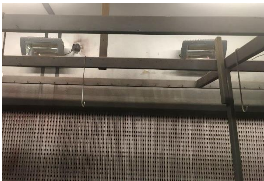
TCS Shipwright ATEX heaters in a spray booth
